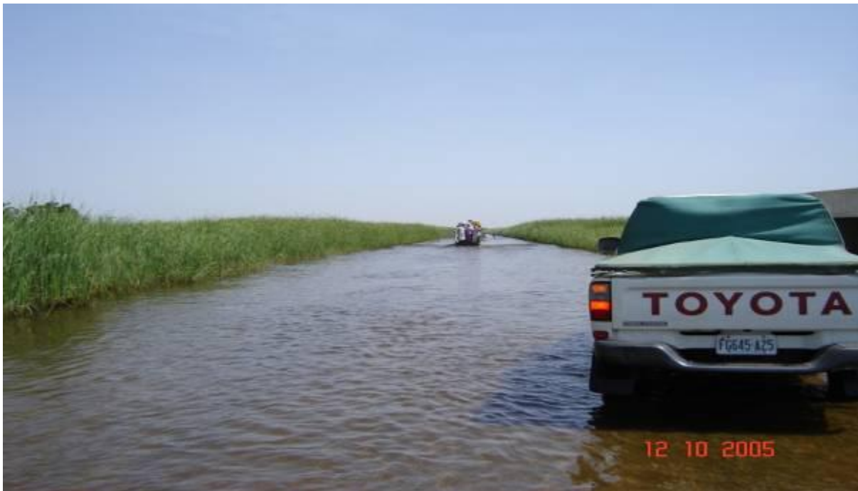
Plate 2: Main road taken over by flood in Nguru Wetland
