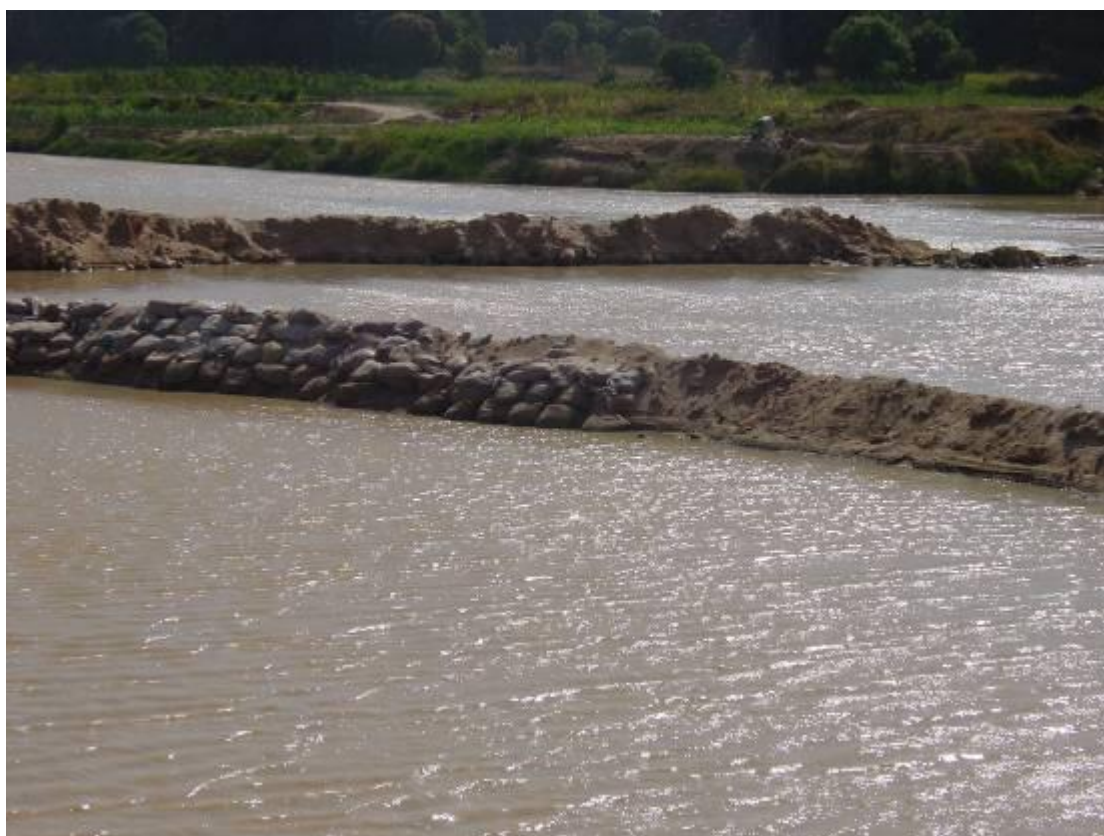
Plate 4: Diversion Structure for KCWS Intake No. 11
